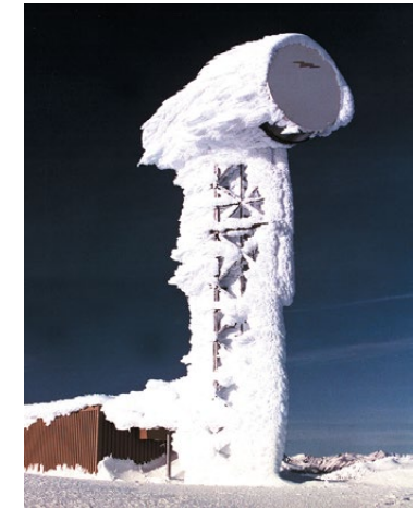
8.15: Ice accumulation on a radome-protected installation
