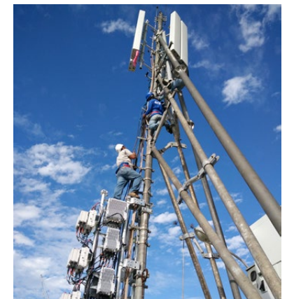
11.13: CommScope network engineering team in the field
