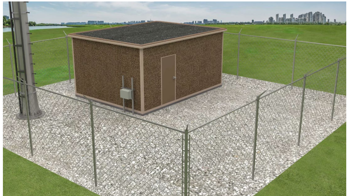
2.5: A traditional cell site enclosure housing radio and base station components
